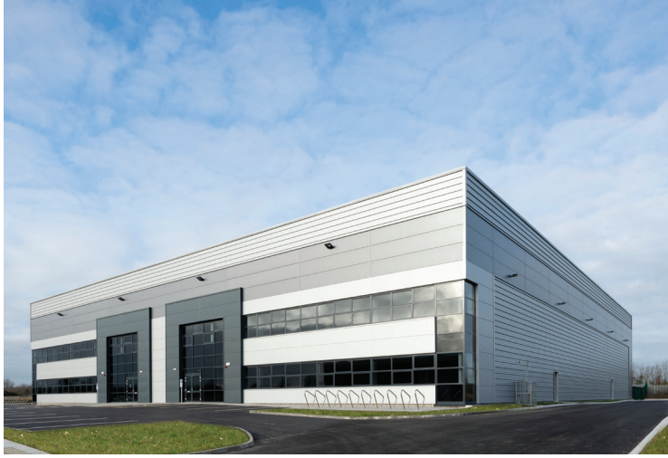
Units A7A & B, North City Business Park, Finglas, Dublin 11 – Let Q3 2020
