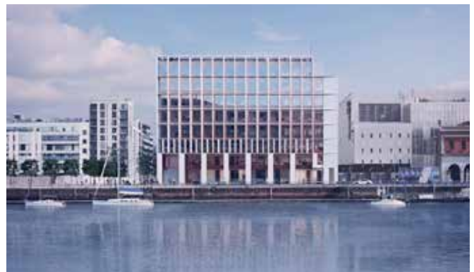
North Wall Quay
