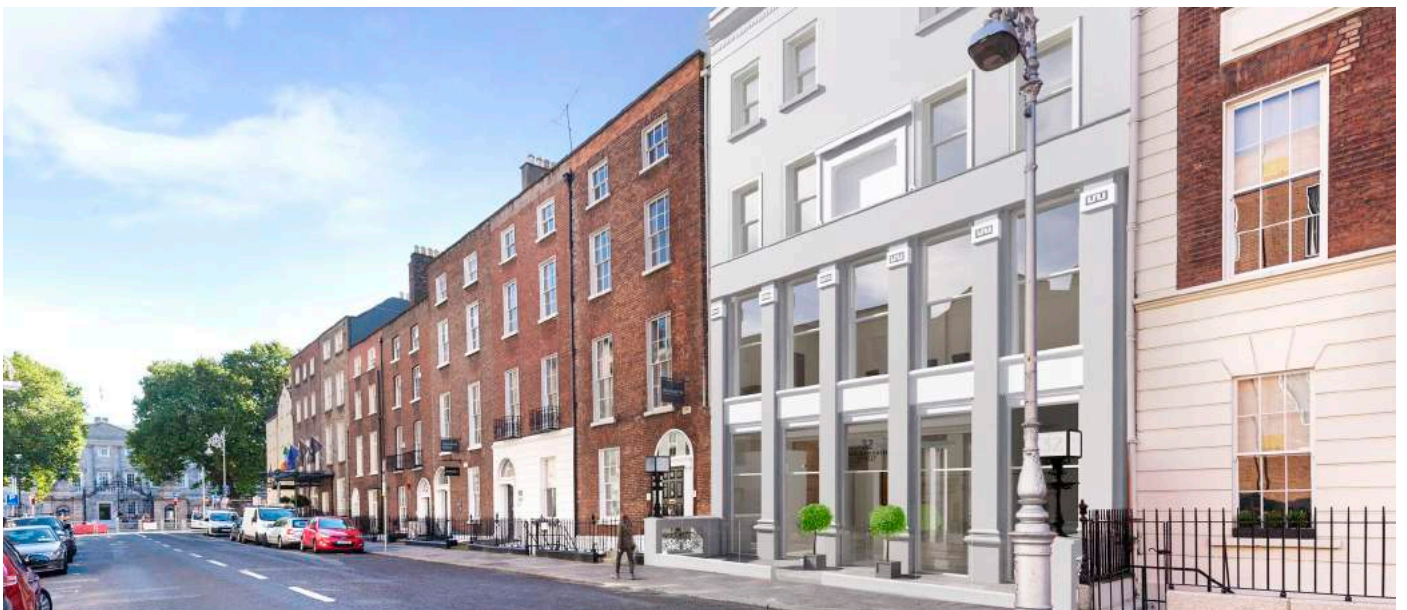
32 Molesworth Street. Recently redeveloped and pre-let by Savills.
