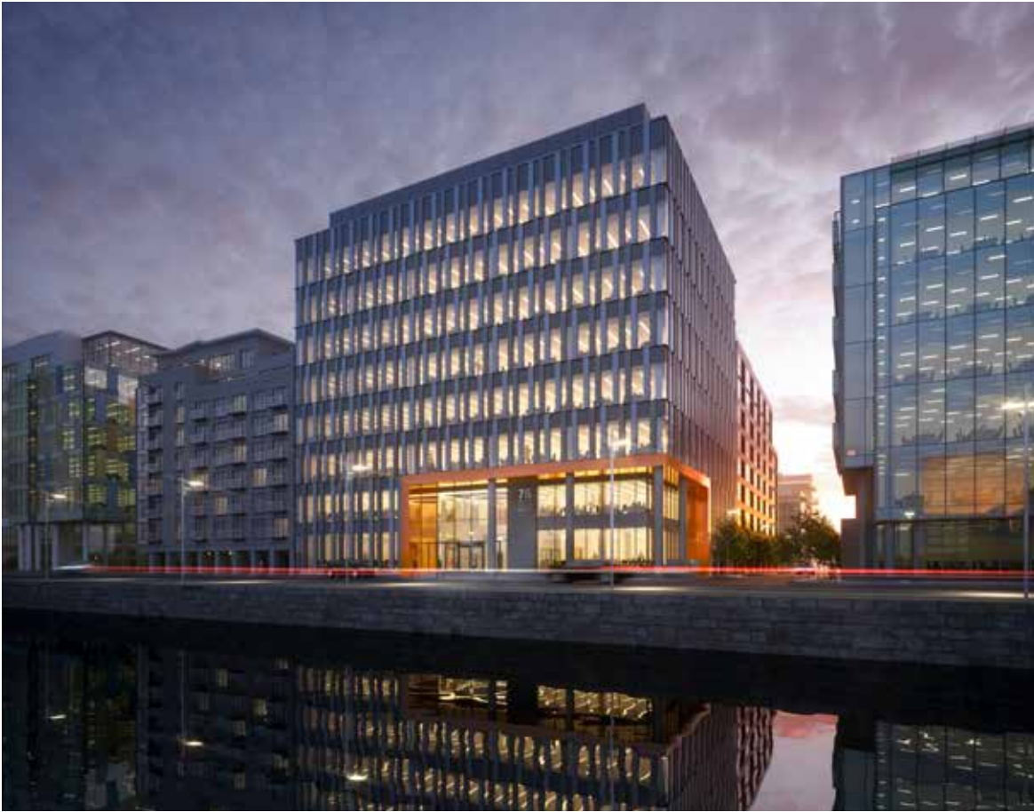
76 Sir John Rogerson's Quay 100,000 sq.ft. of Grade A office HQ space with undisturbed river fronting views available in Q4 2019
