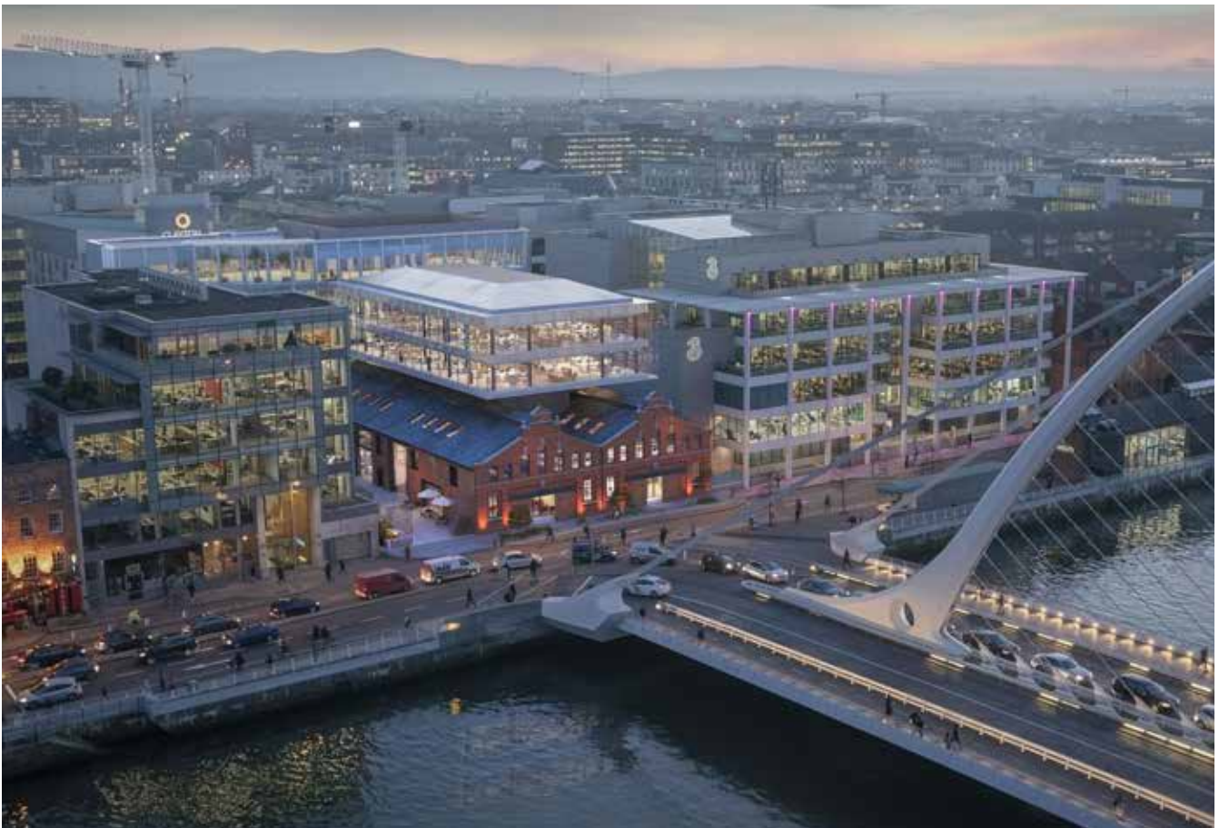
The Tropical Fruit Warehouse, 80,000 sq ft of exceptional office space delivering in Q2 2021
