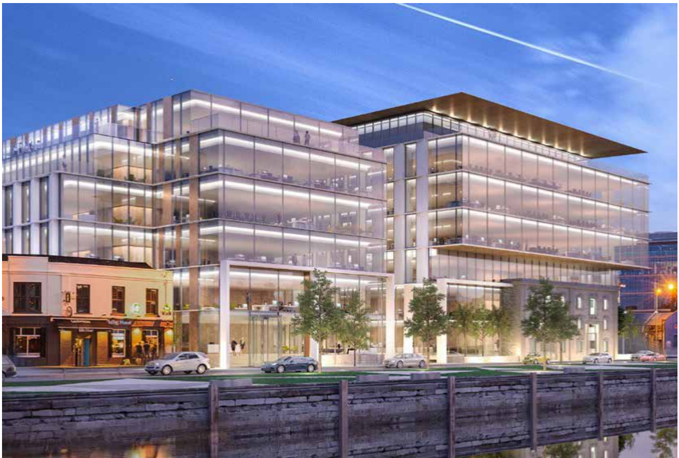
Navigation Square Cork. High quality new office development. Available now.
