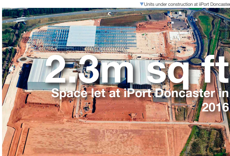
▼ Units under construction at iPort Doncaster
