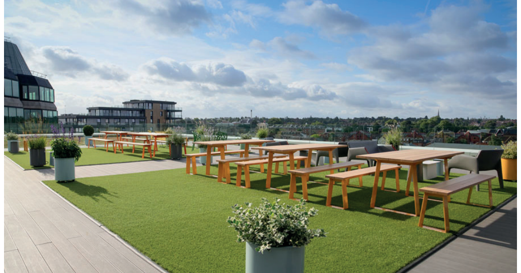
The White Building, Reading has a 3,143 sq ft communal roof terrace
