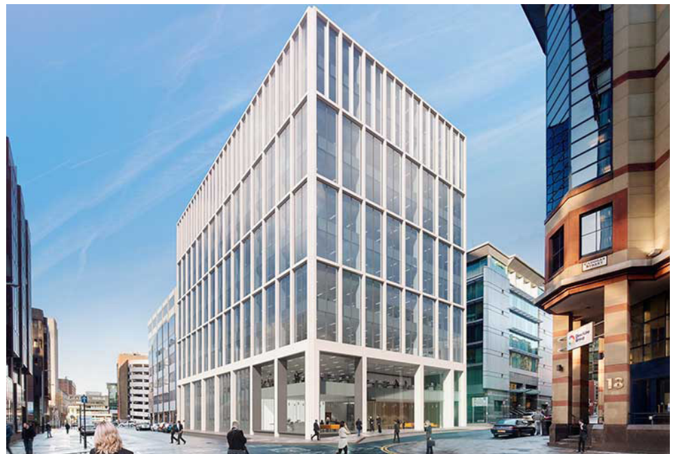
FORE Partnership's Cadworks, above, marks Glasgow's first speculative development since 2015 which will provide 94,000 sq ft of Grade A space on its completion in 2020.
