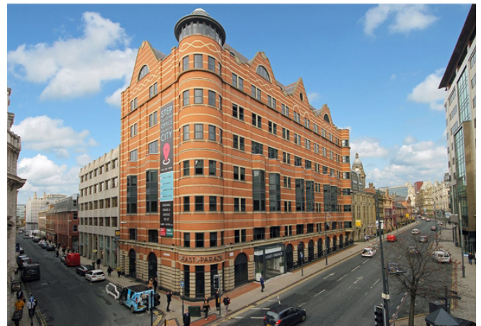
1 East Parade, above, was acquired by Schroders and provides 14,000 sq ft of refurbished space.
