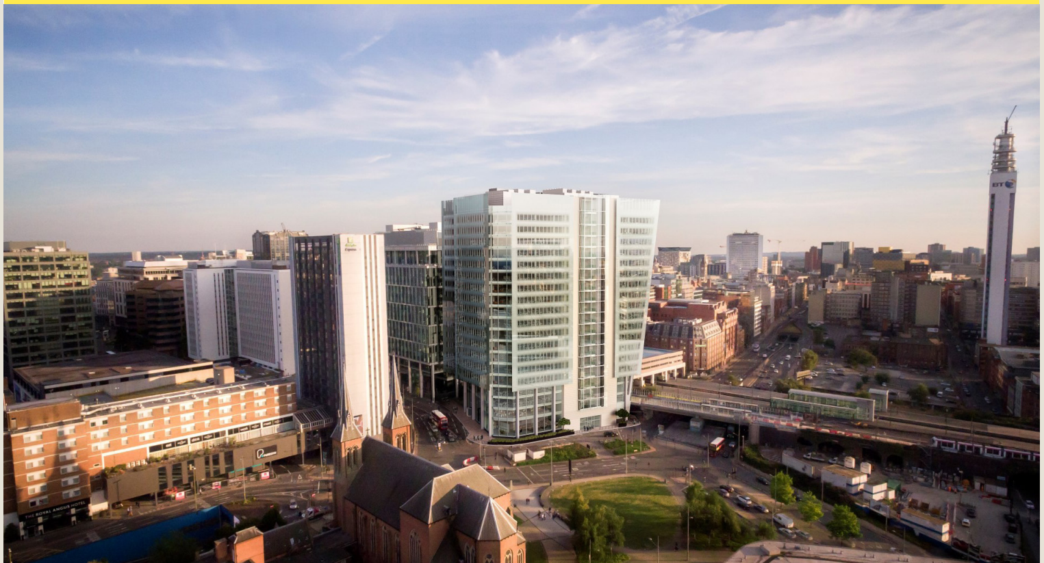
Three Snowhill, Birmingham. 420,000 sq ft under construction set for delivery in 2019.
