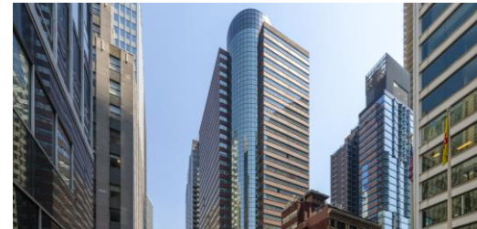
175 Water Street WSA Waterfront LLC
